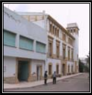
IRTA Research Centre Headquarters, Reus
