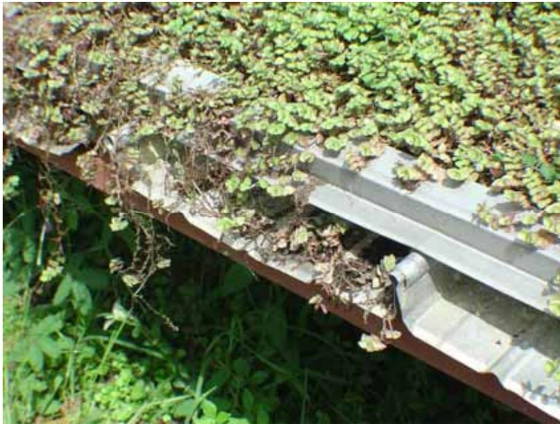
*Singapore trial of extensive system retro-fitted over metal deck*
